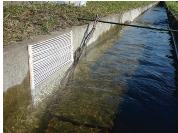
Fig. Structure to give frogs the ability to escape from an agricultural canal.
