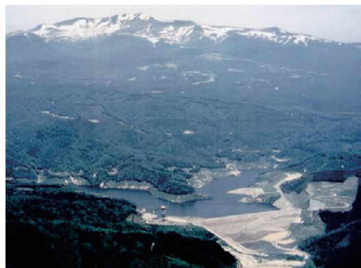
Fig. 21 荒砥沢ダム Overall view of Aratozawa Dam
