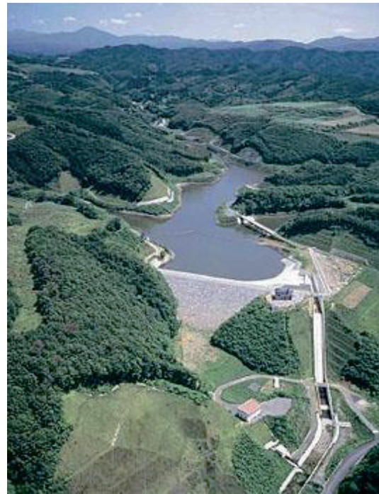
Fig. 54 相川ダム Overall view of Aikawa Dam
