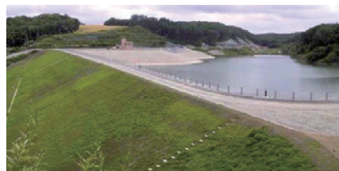
Fig. 9 幕別ダム Overall view of Makubetsu Dam
