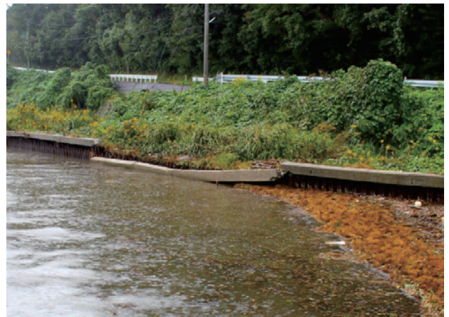
Fig.11 矢板護岸の破壊（石川県） Collapse of embankment of sheet piles (Fukushima prefecture)
