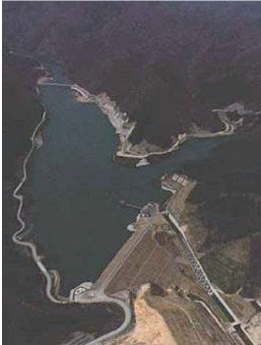
Fig. 38 葛丸ダム Overall view of Kuzumaru Dam
