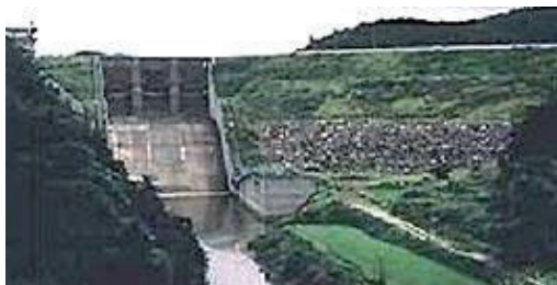
Fig. 66 千五沢ダム Overall view of Sennegosawa Dam
