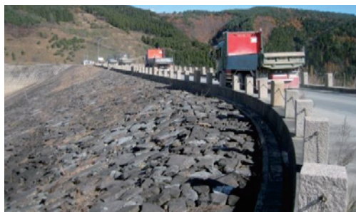
Fig. 25 流入土砂排土運搬用のダンプカー Dump truck for excavation on the crest of Aratozawa Dam
