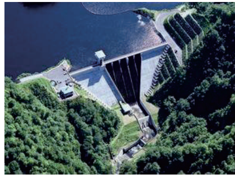
Fig. 56 岩堂沢ダム Overall view of Ganndouzawa Dam
