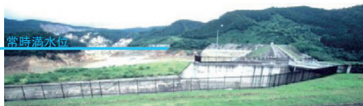
Fig. 23 貯水池越しの左岸上流地山の山体崩壊 Destructed area by landslide over reservoir of Aratozawa Dam
