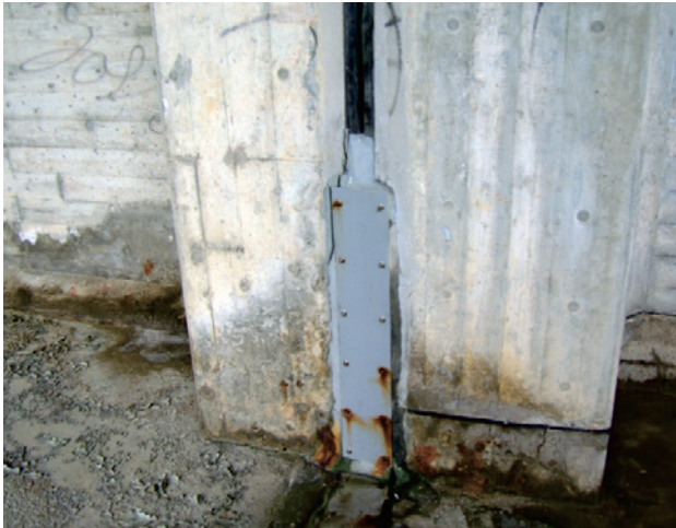
Fig.5 海岸堤防と樋門の継ぎ目補修 (熊本県) Repair of a gap between a coastal dyke and a base of sluices by a filling plate (Kumamoto prefecture)
