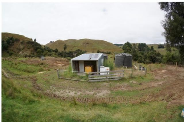
Photo 3.5.3 Water supply pump in Hill country: Water is pumped up from the bottom of valley to the tank at summit of hill with a 200-meter difference of altitude by generator, and supply each paddock.
