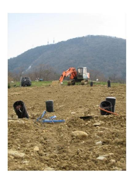
Two pipes are buried for the test of optimizing the size of heat exchanger. (0.3m diameter, 25m long, each buried in the depth of 1.5m and 3m)
