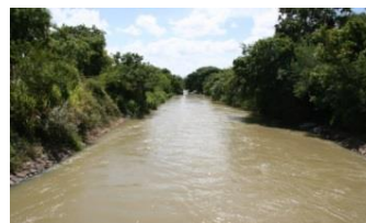
Modern irrigation system
