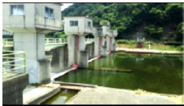
Photo 1: Head work (provided by Kokusai Kogyo Co., Ltd.)
