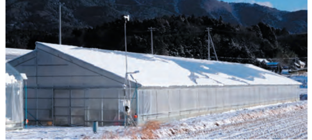
The greenhouse developed in the research can be built at a low cost from mass-produced scaffold materials, making a sturdy structure.
