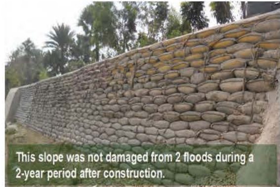
Fig. Rehabilitation work for a rural road embankment in Bangladesh
