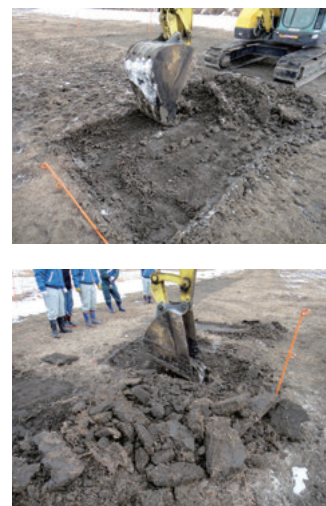
Photo. Soil stripping by the proposed method (upper) and a traditional method (lower).
