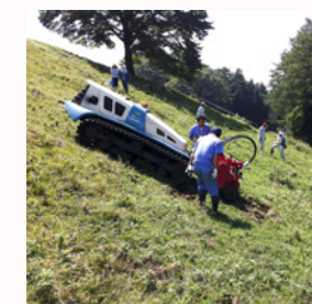
Decontamination on steep slope grassland by a radio-controlled tractor.
