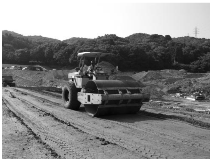
Fig.15 振動ローラによる転圧状況 Compaction of initial-stabilized soil by vibrating roller
