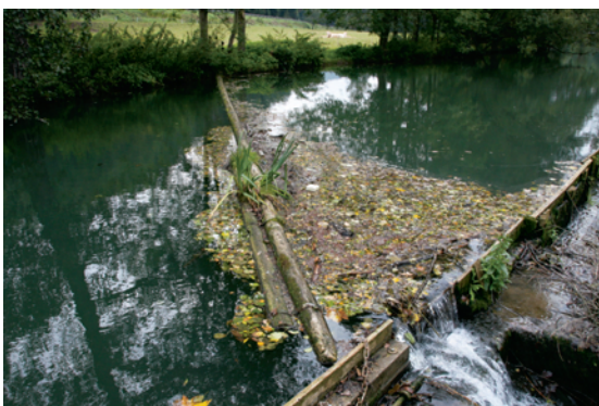
Fig.8 浮遊性ゴミ流入防止板 Board that prevents floating waste from flowing into a sluiceway
