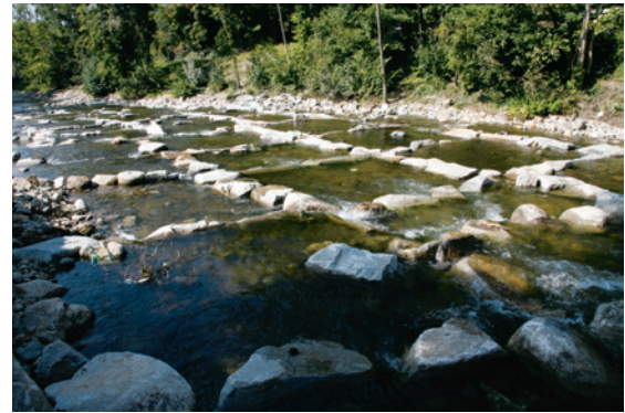
Fig.6 水車設置に伴って環境に配慮した河川改修 River improvement that considers environment along with water mill installation
