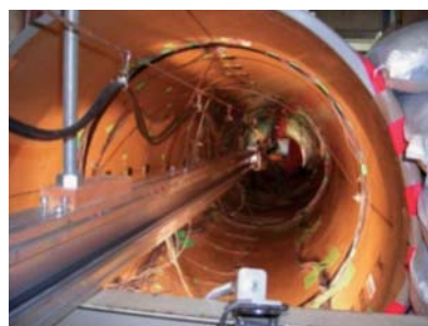
■ Pipeline traffic-loading test
