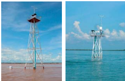
■ Hydro-meteorological observation systems in Tonle Sap Lake
