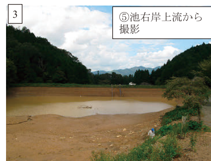
Fig. 18 ⑤池貯水池内の堆砂状況 Sand and mud flowed into ⑤ ike
