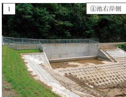
Fig. 16 ④池の洪水吐 Spillway of ④ ike
