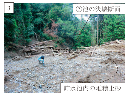
Fig. 23 ⑦池の貯水池内の流入土砂 Sand and wood flowed into ⑦ ike
