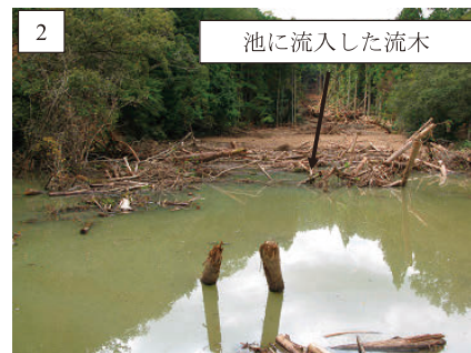
Fig. 6 ①池の貯水池内に流入した土砂 Sand and wood flowed into ① ike
