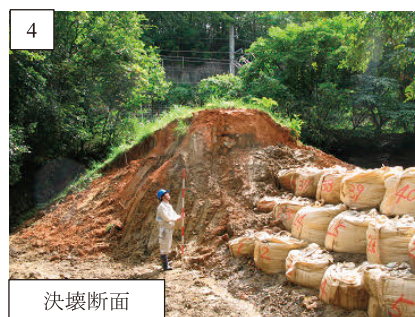
Fig. 9 ②池の決壊断面 Cross section of failure part at ② ike
