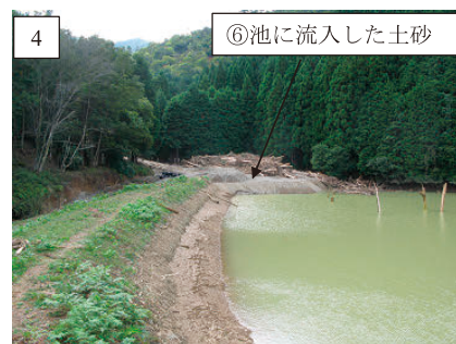
Fig. 19 ⑥池上流部の状況 Upstream of ⑥ ike
