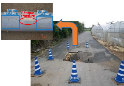
■ Identification of causes in pipeline rupture accidents
