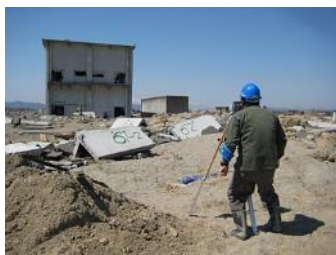
■ On-site survey of tsunami damage
