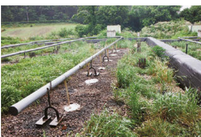
An organic sewage water purification test utilizing constructed wetland
