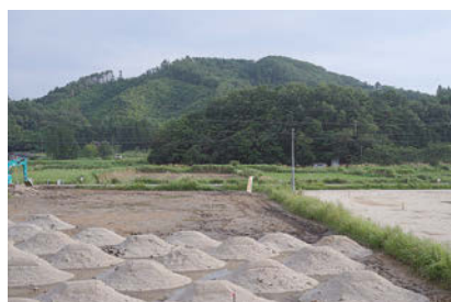
Soil dressing was performed after removal of the topsoil
