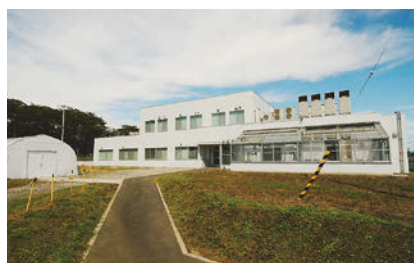
Radioactive substances analysis building (completed in April 2013)
