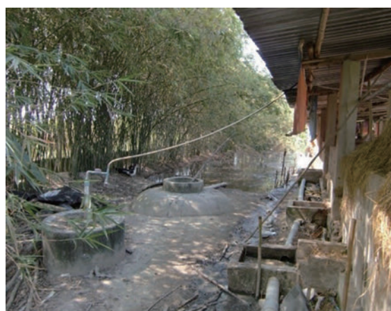
Fig. 7 Biogas digester in a pig farm
