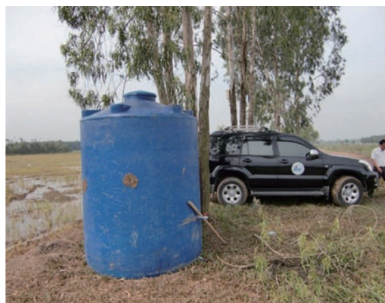
Fig. 8 Storage tank of digested slurry
