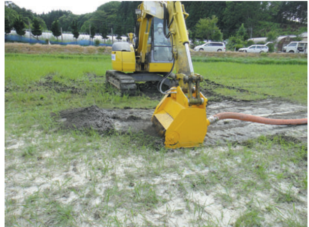
Fig. Removing radioactively contaminated topsoil by a newly developed method
