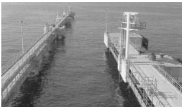
Fig.2 港湾施設の例 Concrete structure of port facility
