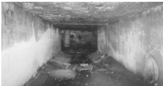
Fig.3 下水道施設の例 Concrete structure of sewerage facility
