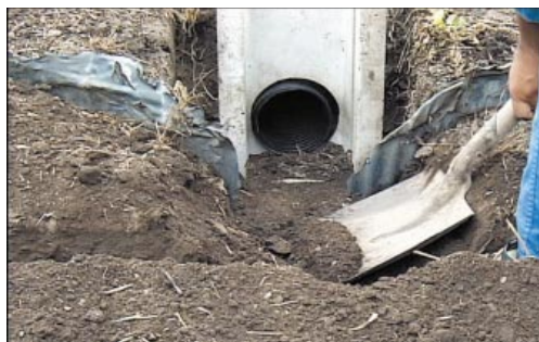
Fig.3 排水マスの敷設替え Drainage box construction
