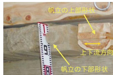
Fig. 9 帆立下部と上部の加工形状 Cutting shape at the upper and lower part of Hotate
