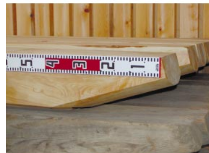
Fig. 8 控の下流端の加工形状 Cutting shape at the lower part of Hikae
