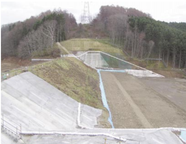
Fig.33 杵臼ダムの既設堤体と嵩上げ予定位置の状況 Upstream view of Kine-usu dam
