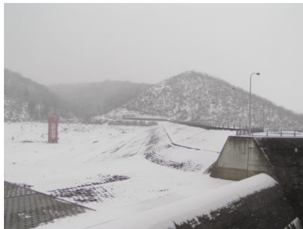
Fig.28 雨煙内ダムの改修後の堤体上流側の状況 Upstream view of Uen-rai dam
