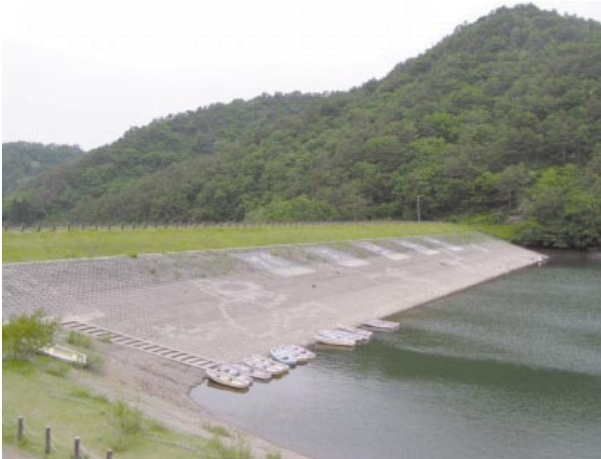
Fig.6 蛭沢ダムの改修事例 Upstream view of Birusawa dam
