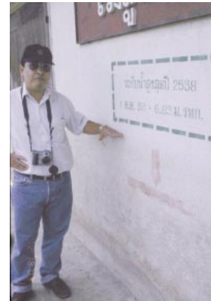
Fig.32-1 バンバン地区北東部揚水機場の小屋外の壁に残されていた洪水時の水位跡 (Fig.21 ) His arm shows 2002 s water level at the flooding. The red line indicates the water level of 1995 s flood central part of this irrigation project region . (puddling term)
