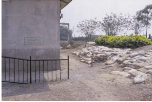
Fig.33-1 別の揚水機場で土嚢を積み上げた跡 ( Fig.21 ) The evidence to pile up sandbags at another pumping station for the 2002 s flood
