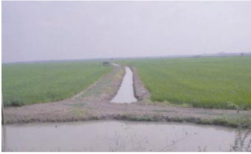
Fig.39 パクハイ地区の堤防近くの乾期水田 ( Fig.21 ) Paddy fields near the bank in dry season
