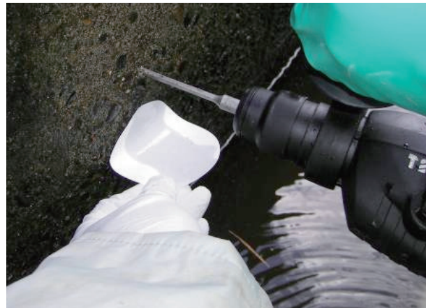
Fig.3 簡易中性化深さ測定 The simple measurement of neutralization
