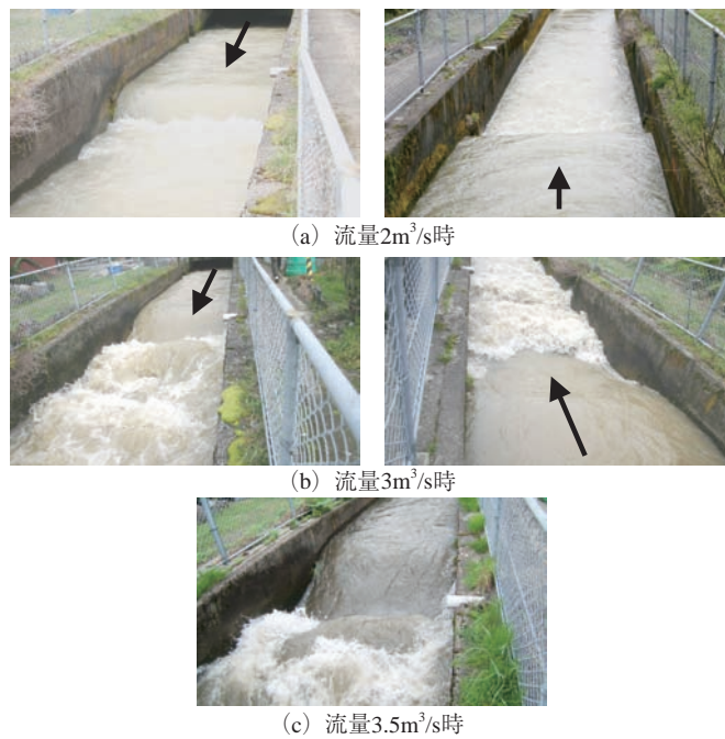
Fig.8 Z号落差工位置の流況 Flow at Zth ground sill
