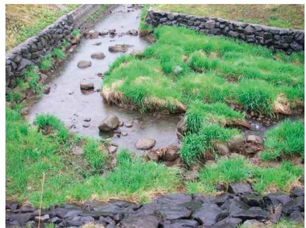
Fig.4 二面張り区間(幅広水路部) Wall lining zone (Widening section)
