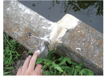
Fig.11 未改修区間のバレル間の横ずれ Wide gap between the barrels of the non-repair section
