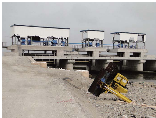
Fig. 97 全景 (牛橋水門) View of the whole structure
