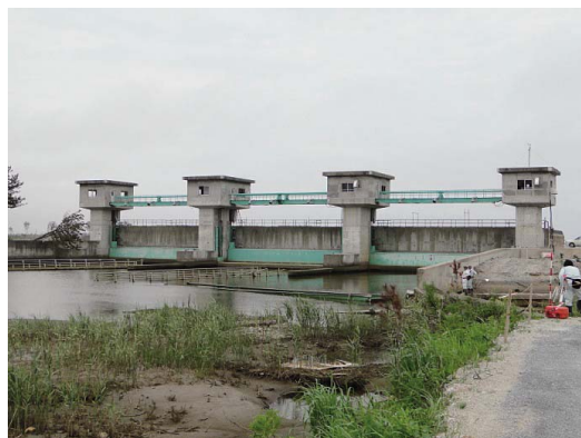
Fig. 102 全景 (坂元水門) View of the whole structure
