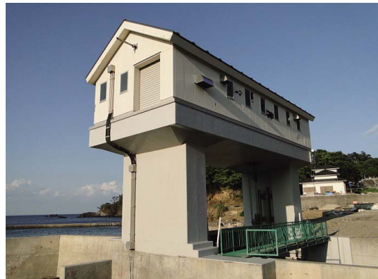
Fig. 84 全景 (長清水川防潮水門) View of the whole structure
