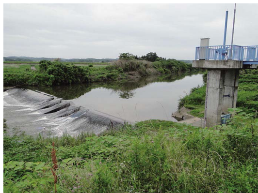
Fig. 39 全景 (行井堂堰) View of the whole structure
