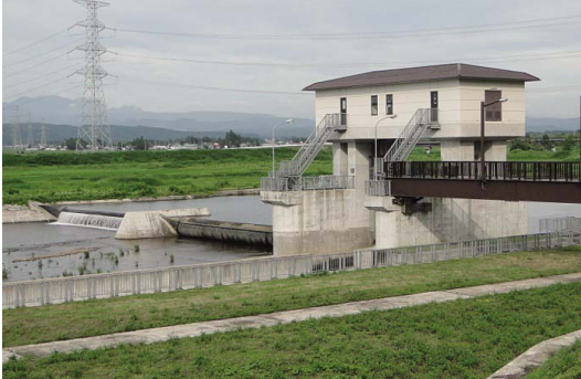
Fig. 64 全景 (館前頭首工) View of the whole structure
