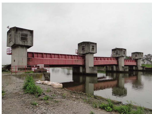
Fig. 94 全景 (貞山堀防潮水門) View of the whole structure
