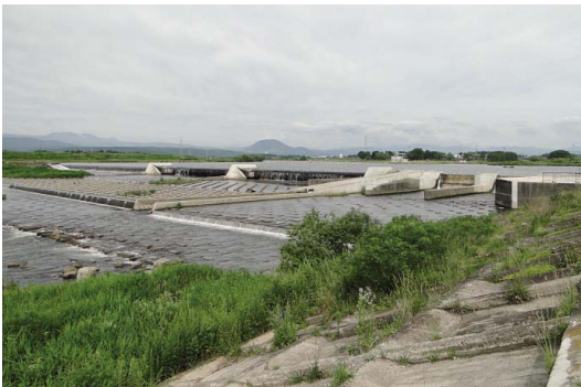
Fig. 65 全景 (上川原頭首工) View of the whole structure
