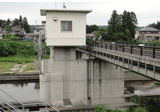
Fig. 66 全景 (大堰) View of the whole structure
