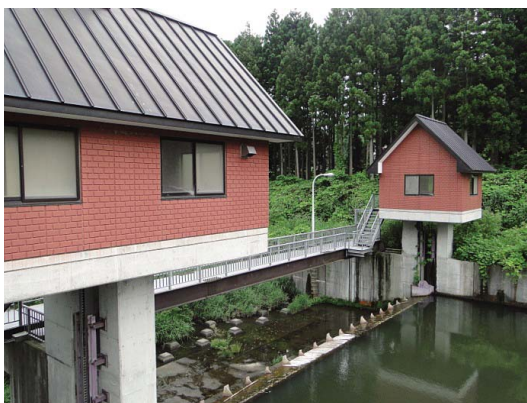
Fig. 29 全景 (川台頭首工) View of the whole structure
