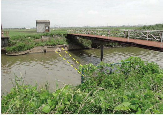
Fig. 53 全景 (矢野目堰) View of the whole structure
