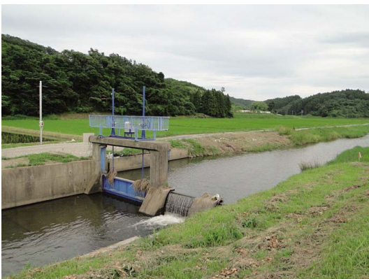
Fig. 42 全景 (幕柳堰) View of the whole structure
