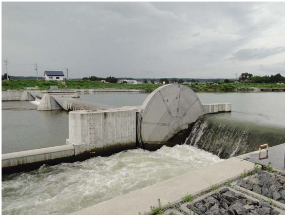
Fig. 28 全景 (秋山頭首工) View of the whole structure
