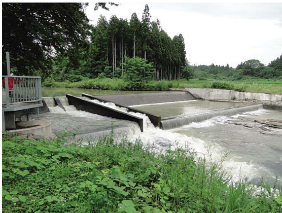
Fig. 19 全景 (岩淵頭首工) View of the whole structure
