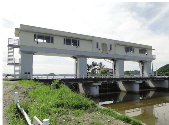
Fig. 91 全景 (東名水門) View of the whole structure
