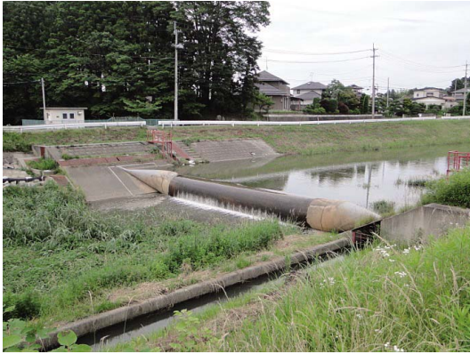
Fig. 40 全景 (山崎堰) View of the whole structure
