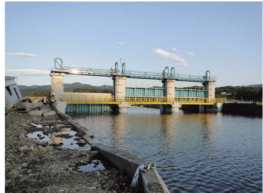
Fig. 78 全景 (折立川防潮水門) View of the whole structure
