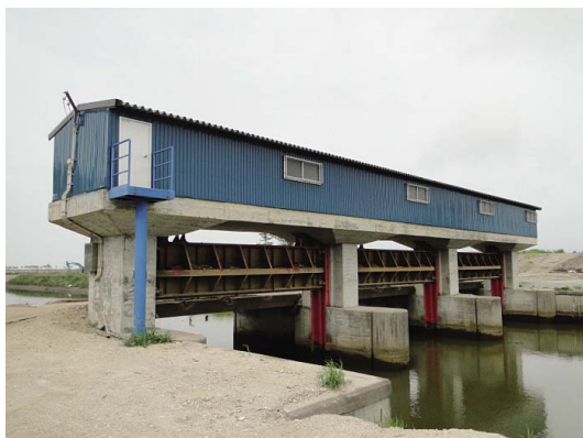
Fig. 100 全景 (高瀬川防潮樋門) View of the whole structure
