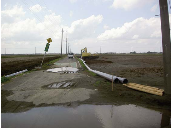
Fig. 44 道路の陥没 Cave-in on the road
