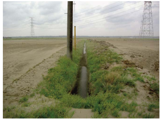
Fig. 77 水田の液状化 Liquefied paddy Occurrence of water leakage
