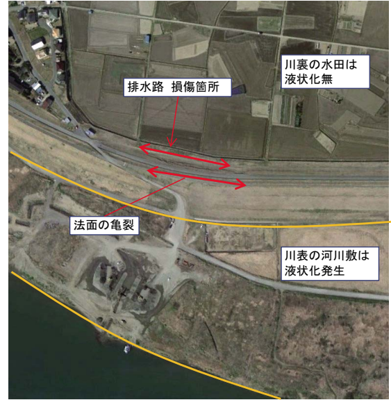
Fig. 47 調査地点 Surveyed sites
