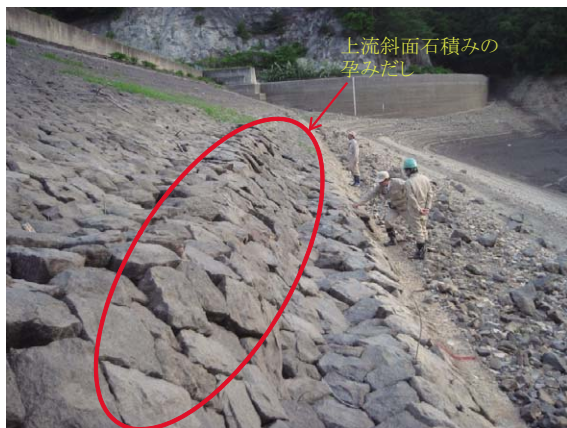
Fig. 10 上流斜面石積みの変形 (上流斜面左岸側より撮影) Deformation of stone protection on the upstream slope (viewed from the left side)
