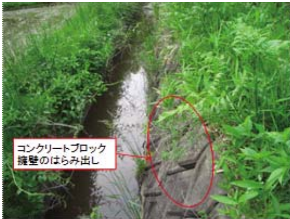
Fig. 27 ミツ池腰石垣の孕み出し Deformation of toe drain blocks of Mitsuike dam
