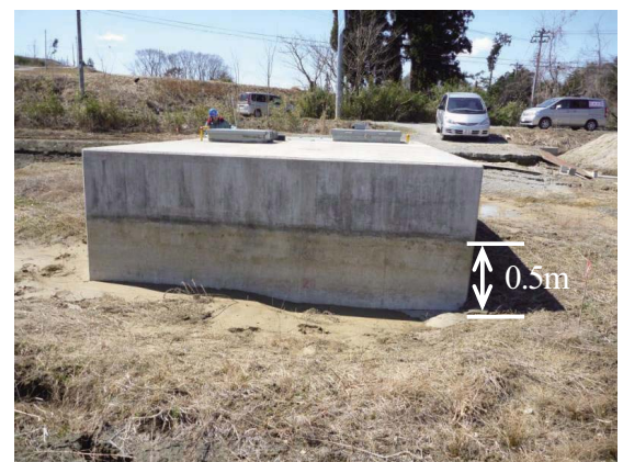
Fig. 27 五本松第1分水工の浮上 Uplift of Gohonmatsu No.1 division works
