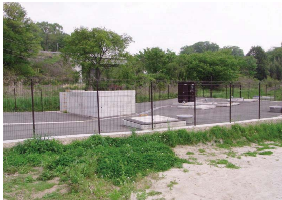
Fig. 29 中畑第1幹線分水工 Nakahata No.1 division works of main line
