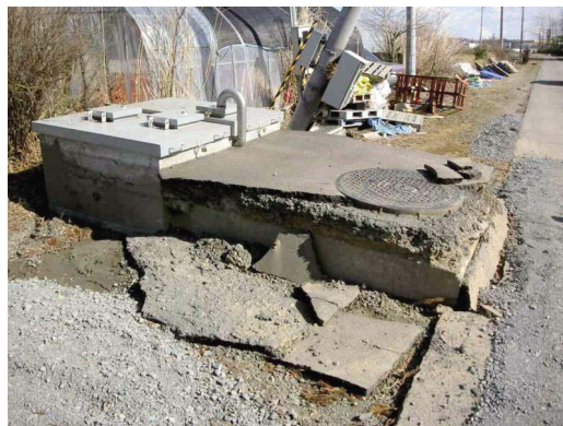
Fig. 54 谷地第 2 分水工の浮上 Uplift of Tanichi No.2 division work
