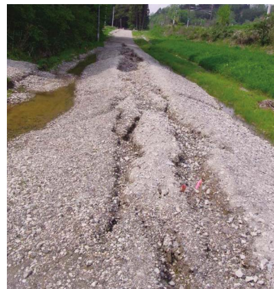
Fig. 32 パイプ敷設道路の亀裂 (矢吹南第2幹線分水工周辺) Cracks on the road around Yabuki Minami No.2 division works
