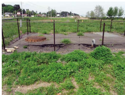
Fig. 56 久来石第 7 空気弁工の路面の亀裂 Cracks on the road surface at Kyuraiishi No.7 air valve
