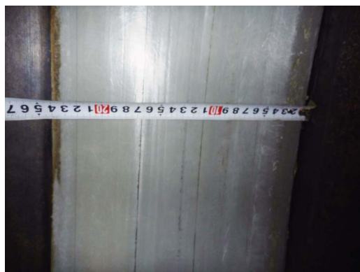
Fig. 55 久来石第 6 空気弁工周辺での継手の抜出し Joint excessive extracted around Kyuraiishi No.6 air valve
