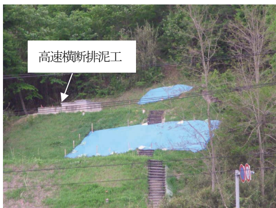
Fig. 25 高速横断排泥工周辺 View around highway crossing blow off
