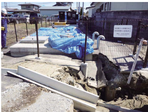
Fig. 39 矢吹第3・4 幹線分水工の被害 Damage to the Yabuki No.3・4 division works of main pipeline
