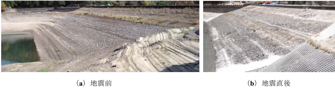
Fig. 49 地震前・後の上流法面 Upstream slope before (left figure) and after (right figure) the earthquake
