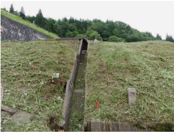
Fig. 20 地区内水路の状況 Situation of channels
