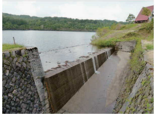
Fig. 38 余水吐の状況 Situation of spillway
