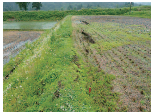
Fig. 23 畦畔法面が滑り田面に発生した亀裂 Cracks of a paddy field with collapse of a levee slope
