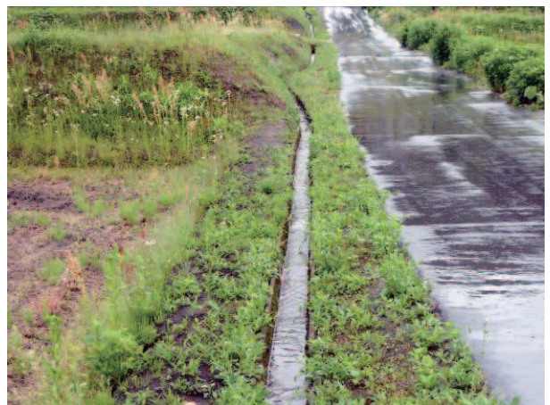
Fig. 29 用水路の状況 Situation of channel
