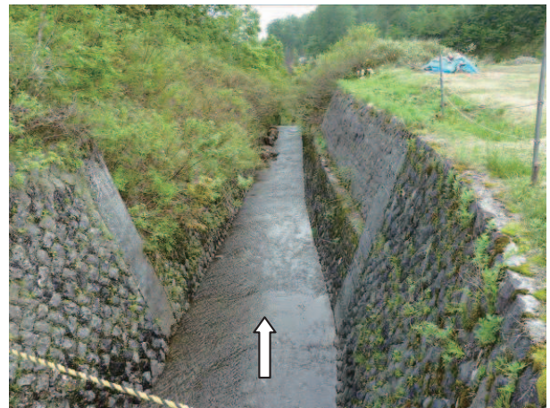
Fig. 39 余水吐放流工の状況 Situation of spillway and discharge
