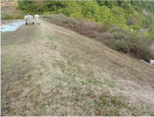
Fig. 41 堤体下流法面 (右岸より) Downstream slope (right side)
