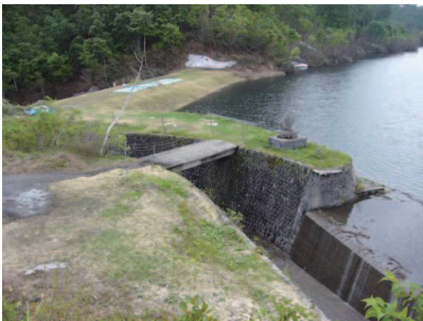
Fig. 36 堤体と余水吐 Earth dam and spillway
