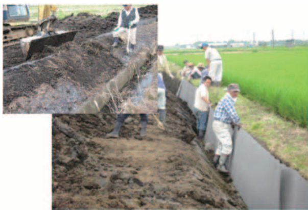
Fig. 21 畦畔際の漏水対策 Leakage control beside levee
