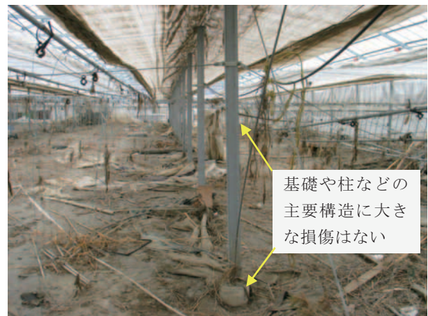
Fig. 23 津波の被害を受けた大屋根型連棟温室 (①) の内部の状況 Internal situation of damaged multi-span greenhouse (No. 1) by the tsunami
