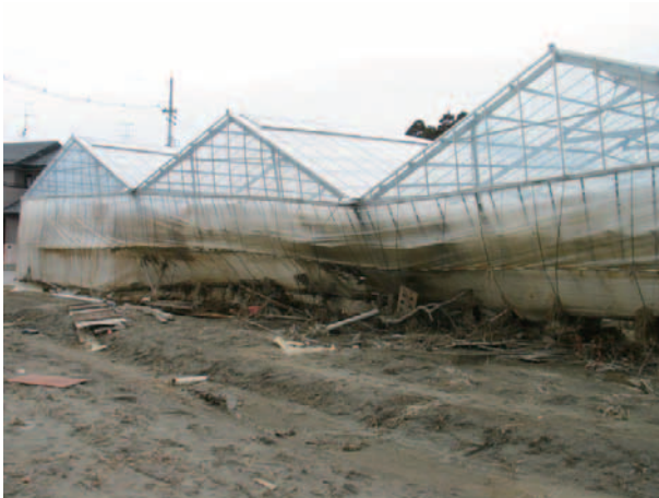
Fig. 20 津波の被害を受けた大屋根型連棟温室 (②) の外部の状況 External situation of damaged multi-span greenhouse (No. 2) by the tsunami
