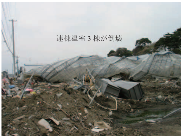
Fig. 27 津波の被害を受けた大屋根型連棟温室の外部の状況 External situation of damaged multi-span greenhouse by the tsunami
