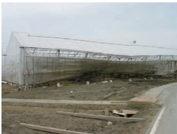
Fig. 19 津波の被害を受けた大屋根型連棟温室 (①) の外部の状況 External situation of damaged multi-span greenhouse (No. 1) by the tsunami
