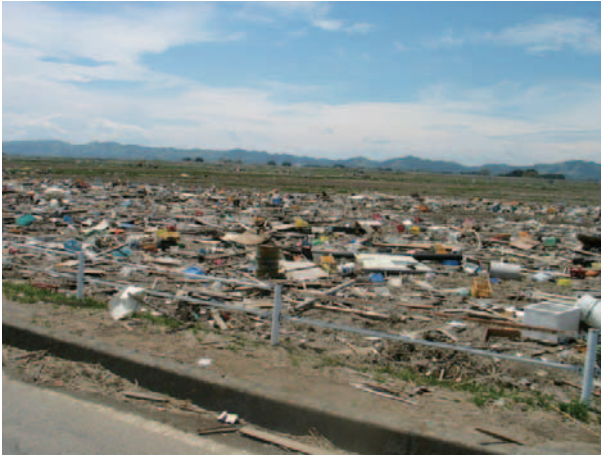
Fig. 2 津波の被害を受けた亙理町荒浜地区の農地の状況 Situation of damaged farmland in Arahama, Watari town by the tsunami
