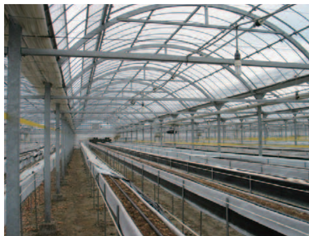
Fig. 5 津波の被害を受けた丸屋根型連棟温室の室内の状況 Internal situation of damaged curvilinear multi-span greenhouse by the tsunami
