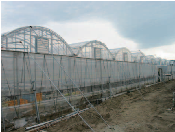
Fig. 4 津波の被害を受けた丸屋根型連棟温室の外部の状況 External situation of damaged curvilinear multi-span greenhouse by the tsunami
