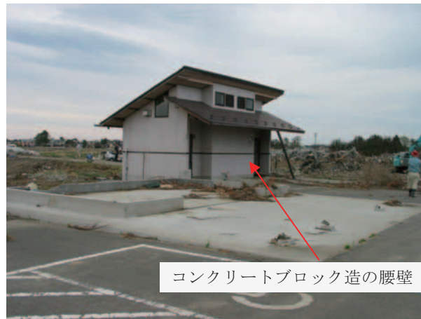
Fig. 15 津波の被害を受けた農産物直売所の状況 Situation of farmer's shop after the tsunami
