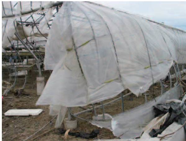
Fig. 9 津波の被害を受けた大屋根型連棟温室（③）の外部の状況 External situation of damaged multi-span greenhouse (No. 3) by the tsunami
