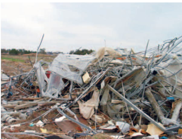
Fig. 13 津波の被害を受けた丸屋根型連棟温室の建設資材 Construction of damaged gothic multi-span greenhouse by the tsunami
