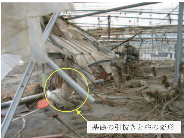
Fig. 22 津波の被害を受けた大屋根型連棟温室 (②) の室内の状況 Internal situation of damaged multi-span greenhouse (No. 2) by the tsunami
