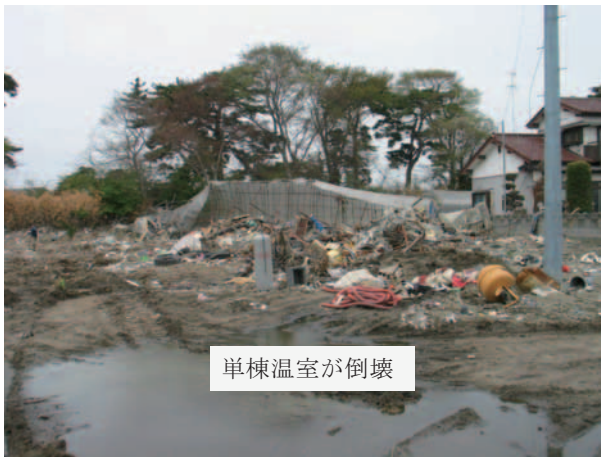
Fig. 29 津波の被害を受けた大屋根型単棟温室の外部の状況 External situation of damaged single-span greenhouse by the tsunami
