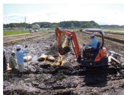
Fig. 13 暗渠排水の施工状況 Installation of subsurface drainage
