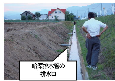
Fig. 7 排水路整備 Drainage channel improvement
