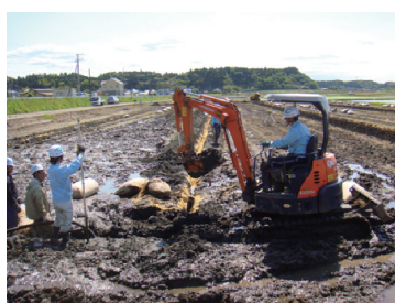
Fig. 6 暗渠排水整備 Subsurface drainage improvement
