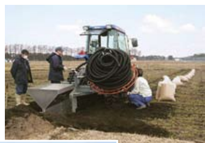
Simplified installation equipment for subsurface drain
