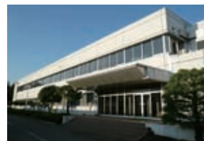
Joint Laboratory Building for the Development of Budding Technologies
