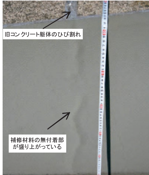
Fig.6 無付着区間の盛り上がり Peeling of the repair material at the section of unbonded area
