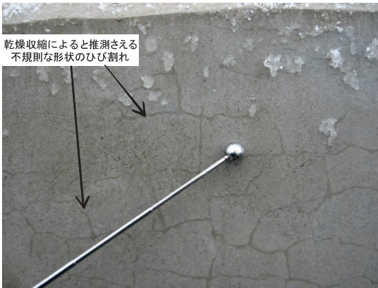
Fig.7 PCMの亀甲状のひび割れ Map Cracking on the surface of PCM
