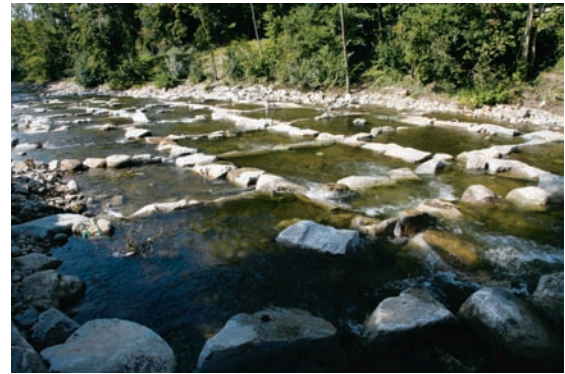
Fig.6 水車設置に伴って環境に配慮した河川改修 River improvement that considers environment along with water mill installation
