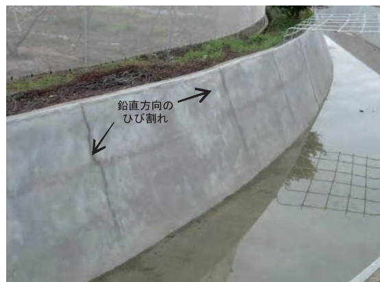
Fig.1 PCMのひび割れ Cracks on the surface of PCM
