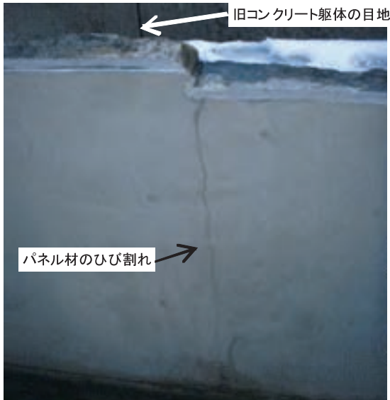
Fig.3 パネル材料のひび割れ Crack on the surface of the organic panel lining material
