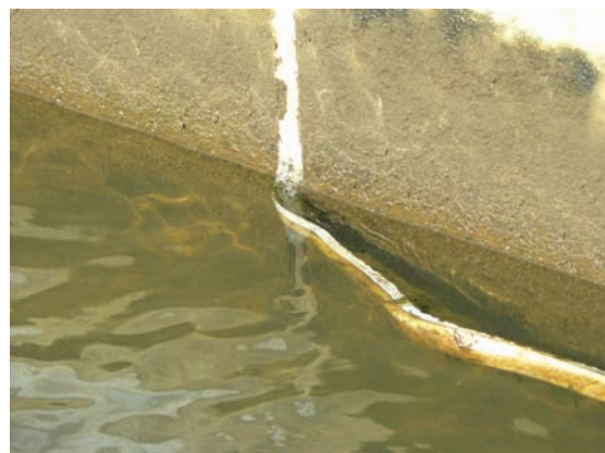
Fig.14 不定形目地材の脱落 Peeling of canal joint sealants
