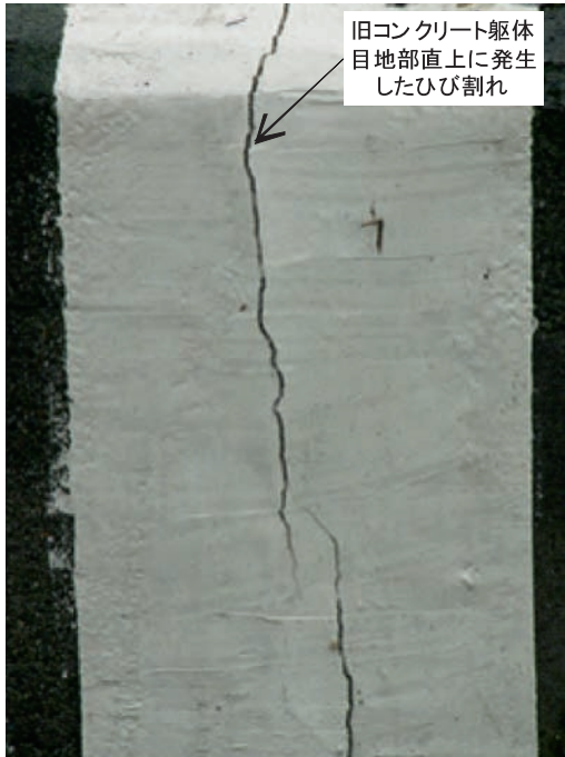
Fig.4 目地補修材料のひび割れ Cracks on the surface of canal joint repair material
