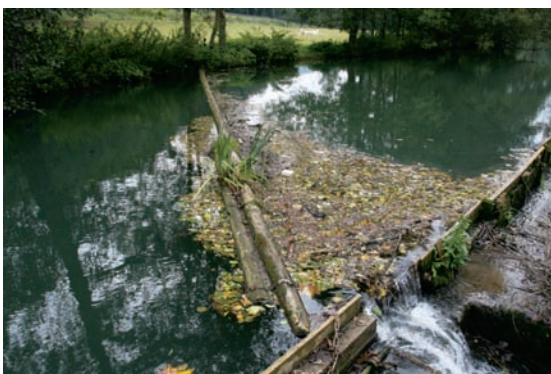
Fig.8 浮遊性ゴミ流入防止板 Board that prevents floating waste from flowing into a sluiceway
