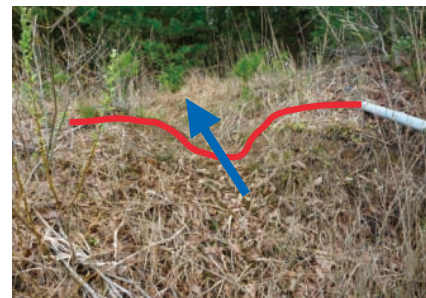
Fig.7 土水路型式の洪水吐 Spillway of earth canal type
