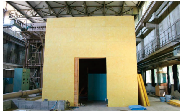
Fig.1 施工中の防音室 Sound proof room under construction
