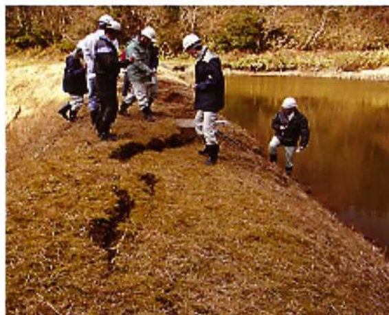
■ Danger diagnosis of the reservoir stricken by the Noto Hanto Earthquake in 2007
