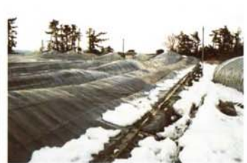
■ Greenhouse damaged by snow load
