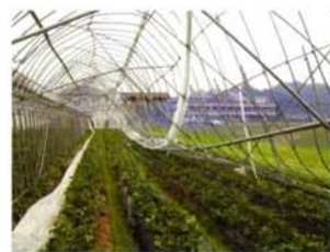
■ Pipehouse damaged by strong wind
