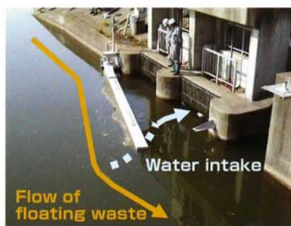
■ Equipment that prevents inflow of floating trash in the sluice gate of head works
