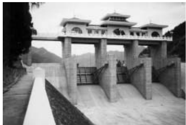
Fig. 59 Three Gates and the Spillway of the Hongjin Dam Rehabilitated in 2001. (September, 2001)
