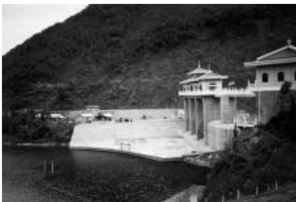
Fig. 58 The Spillway of the Hongjin Dam in Zhejiang Province Rehabilitated in 2001. (September, 2001)
