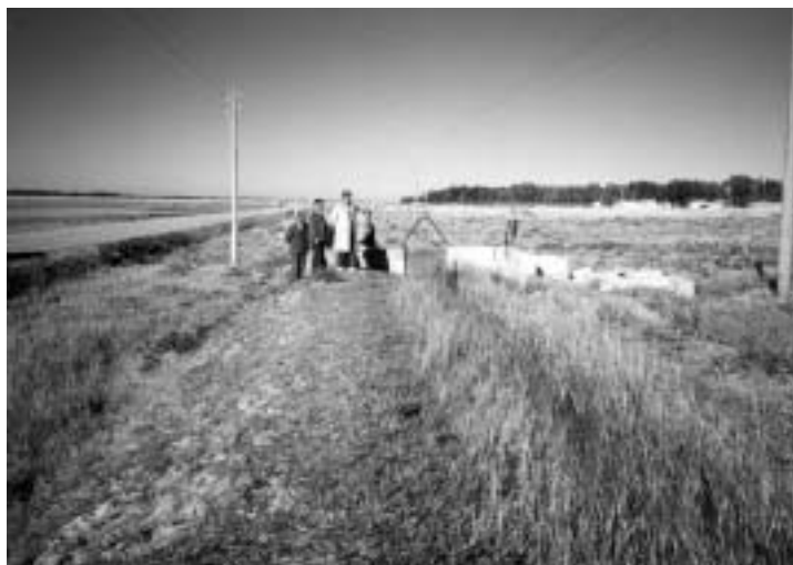
Fig. 45 A Canal Lining in Gansu Province - Consisting of Plastic Film, Sand and Grass. (October, 1995)
