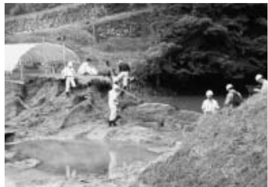
Photo 5-2 大谷ため池の決壊状況 (左岸下流側より撮影) Condition of Ootani dam breach (viewed from downstream)
