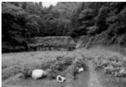
Photo 3-1 迫の益ため池の決壊状況（下流側より望む） Breached Sakonoeki dam (viewed from downstream)
