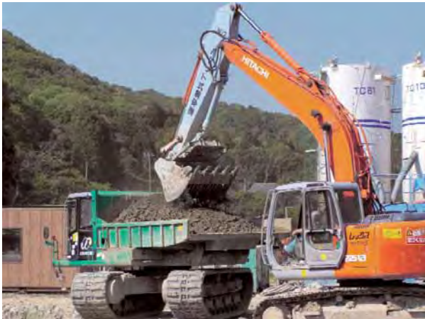
Photo.5 初期固化土の解砕・積込み状況 (バケット式解砕機) Crushing of initial-stabilized soil by bucket type crusher
