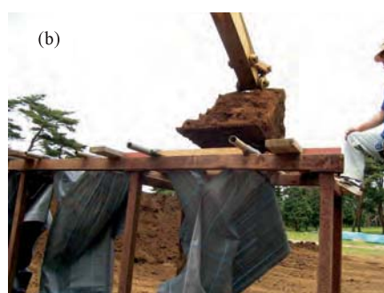
Procedure for making soil bags with a screw extruder: (a) backhoe with the screw extrusion device; (b) Infilling recycle concrete aggregates into the geosynthetic soil bags
