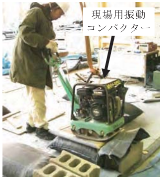
Fig. 185 土嚢の予備転圧状況 Pre-compaction of soil bag
