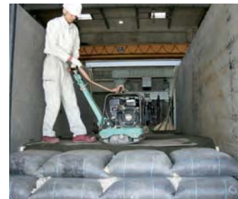
Fig. 188 堤体土の締固め状況 Compaction of backfill material
