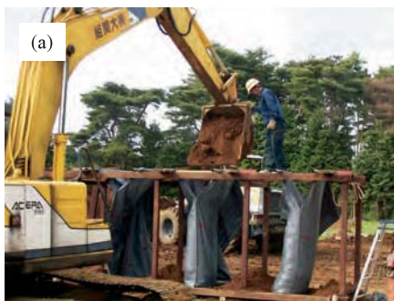
Procedure for making soil bags with a screw extruder: (a) backhoe with the screw extrusion device; (b) Infilling recycle concrete aggregates into the geosynthetic soil bags
