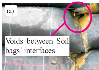
Fig. 236 軽微な損傷: (a) 土嚢積層斜面背面のサヤ土が吸い出された痕跡; (b) 土嚢材の摩耗とパンチング穴 Minor or moderate damages: (a) evidence of sucked backfill materials from cell zone through the voids between soil bag interfaces; (b) attrition surface and perforations on soil bag surface
