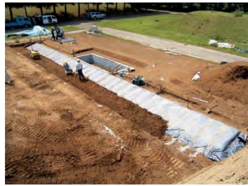
Fig. 264 土嚢背面に裏込め材を巻き出した状況 Backfilling behind soil bags stacked on the slope
