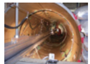
Traffic loading test of pipeline
