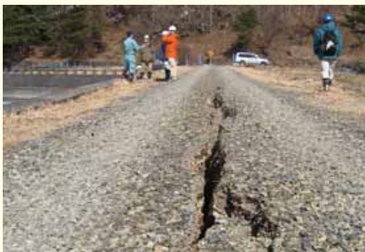
Diagnosis of degree of hazards in storage reservoir affected by the Great East Japan Earthquake
