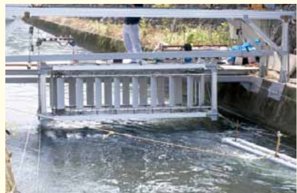
A water wheel for micro hydro power generation installed in irrigation channel
