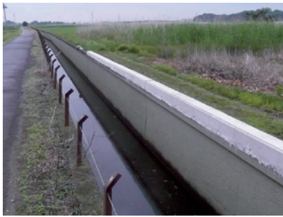
Fig.16 溢水が生じた区間の嵩上げ補修状況 The expansion of canals walls on the section where overflow occurred
