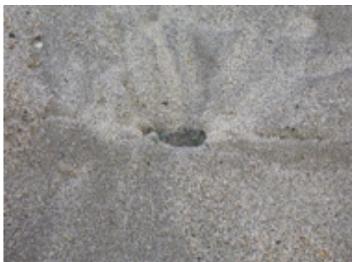
Fig.10 噴出砂の痕跡 Sand flow around seawall
