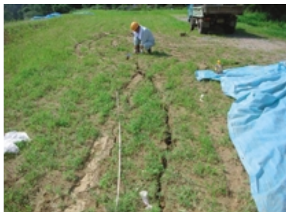
Fig.23 右岸天端の亀裂（大池） Continuous cracking on the top of a dike
