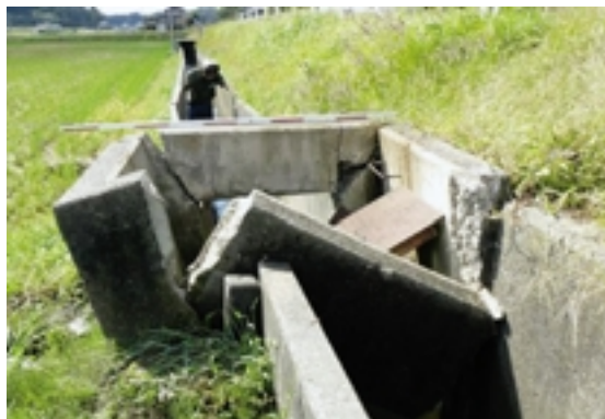
Fig.44 水路脇法面の押し出しによる分水柵の破損 Damage to a diversion device by sideways pressure from the upslope direction
