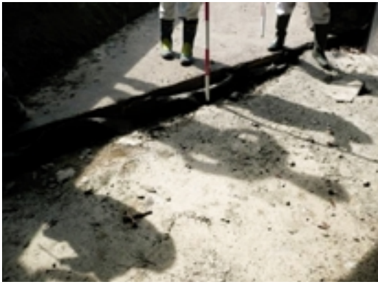
Fig.11 もたれ擁壁水路における底版の段差 Raised hump in floor of concrete canal retaining wall
