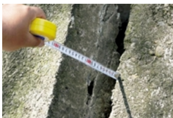
Fig.10 もたれ擁壁水路側壁における目地のずれ・開き Tilting and expansion of a joint in a canal retaining wall
