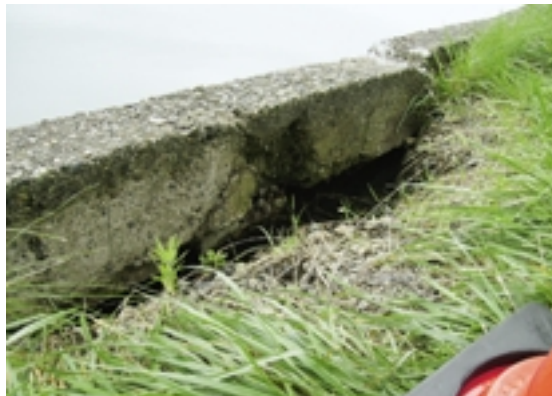
Fig.40 護岸壁の破損（坂田池） Damage to a revetment wall
