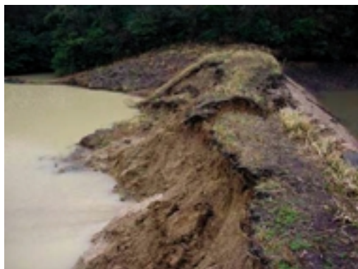
Fig.4 平田池の上流斜面の崩壊状況 (平田池) Slip failure on the upstream slope
