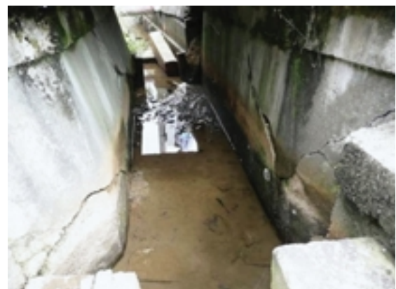
Fig.51 水路暗渠部側壁のひび割れ Cracking in the sidewalls of a culvert
