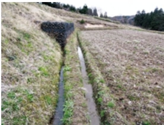
Fig.8 布団籠の設置状況 Installation of a basket filled with stones
