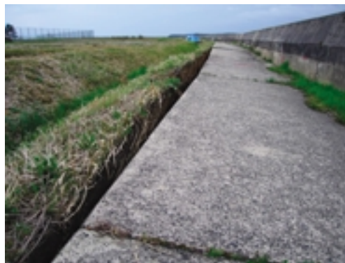
Fig.7 隣接する地盤の沈下 Settlement of backfill foundation
