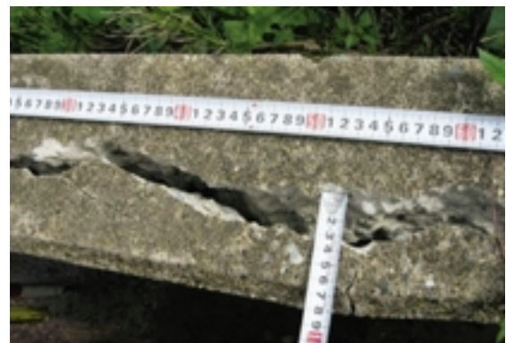
Fig.4 止水板延長上に延びるひび割れ Crack in a concrete water stop
