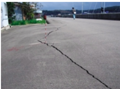
Fig.8 控え杭の突出（地盤の沈下，小牧地区） Settlement of foundation around pile
