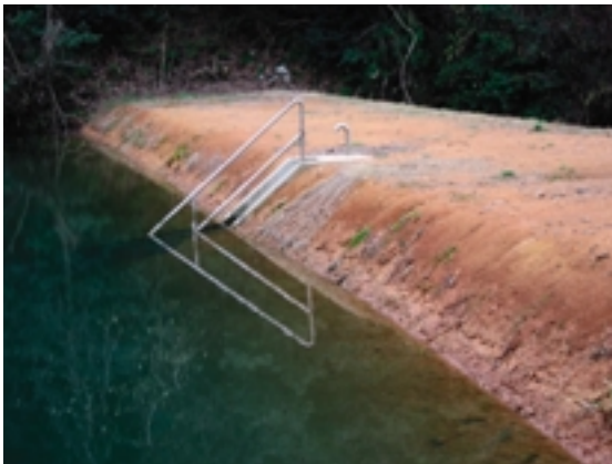
Fig.16 斜樋部分の崩壊 Slope failure at the inlet works
