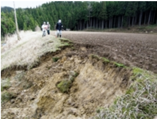
Fig.4 用水路への土砂流入 Inflow of earth and sand into an irrigation
