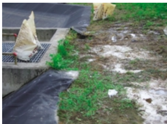
Fig.10 取水口天端の沈下（柿木第 6-1 号 FP） Settlement of embankment around out let box
