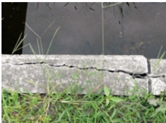
Fig.31 側壁天端止水板から延びるひび割れ Crack in a water stop at the crest of a canal
