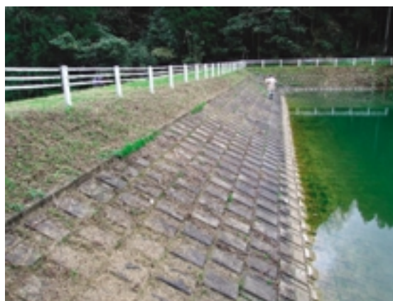
Fig.12 上流法面保護ブロックの沈下 Settlement of the concrete block mat on the upstream slope
