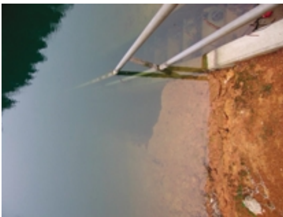
Fig.17 斜樋周辺堤体の崩壊 Slip failure of the slope at the inlet work
