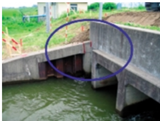
Fig. 50 排水樋門と矢板護岸工取り付け部からの漏水 Leakage from a joint between a sluice gate and sheet-pile
