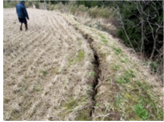
Fig.3 畦畔際の亀裂 Fissure along a levee
