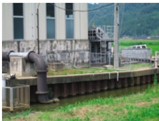
Fig. 52 建屋周辺地盤の沈下 Settlement of ground around a building
