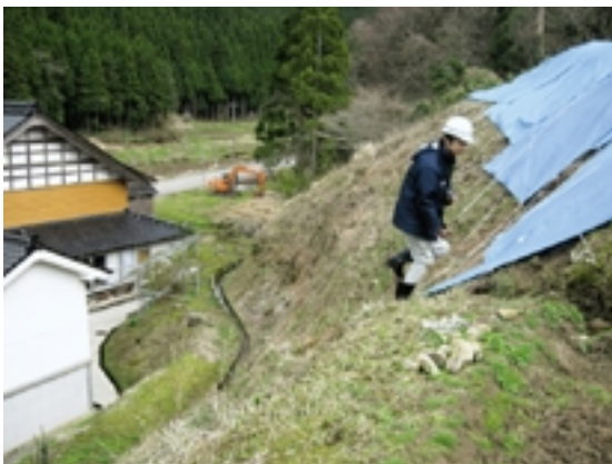
Fig.5 法面の亀裂と法下の家屋 Fissures on a slope with houses below the slope
