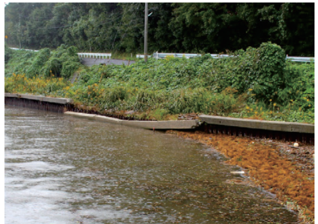
Fig.11 矢板護岸の破壊（石川県） Collapse of embankment of sheet piles (Fukushima prefecture)
