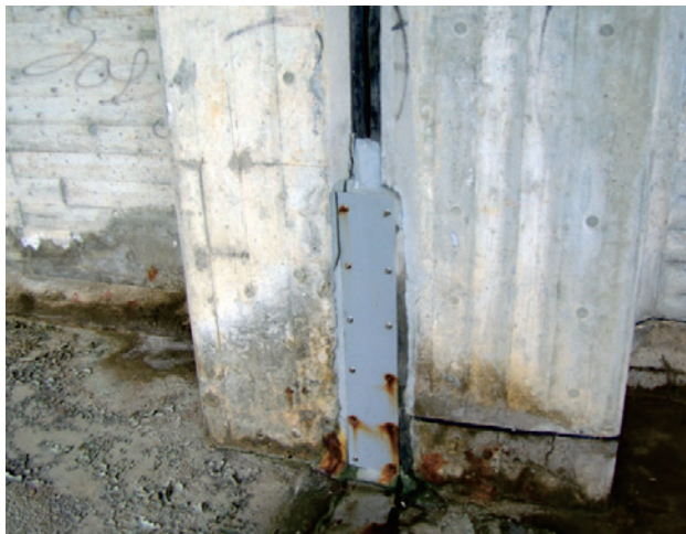
Fig.5 海岸堤防と樋門の継ぎ目補修 (熊本県) Repair of a gap between a coastal dyke and a base of sluices by a filling plate (Kumamoto prefecture)
